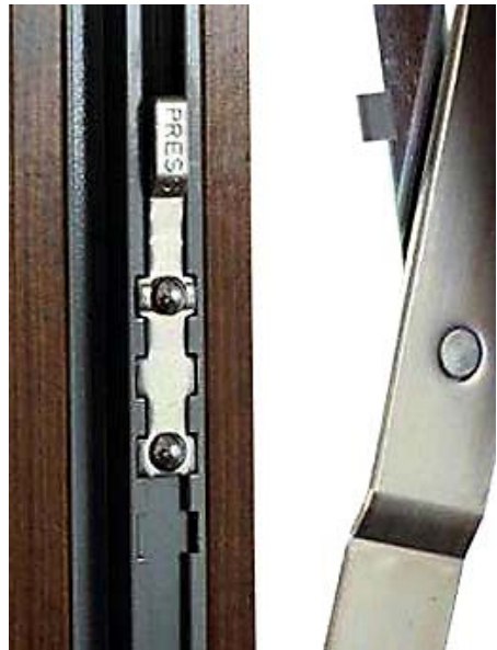
Figure 1.7. Catcher for an SW14 top swing window
